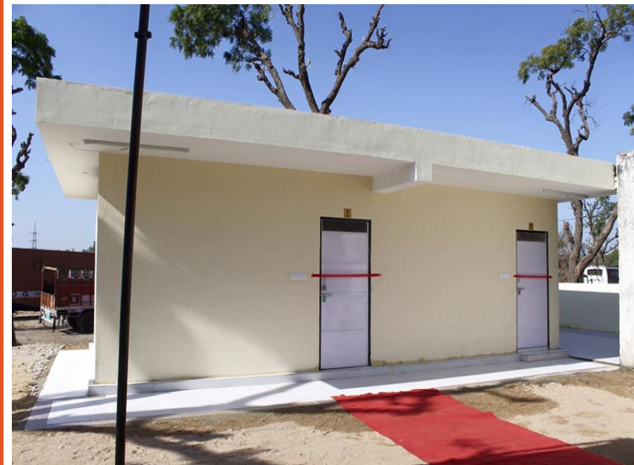
Toilet Block at Bagru Police Station, Jaipur
