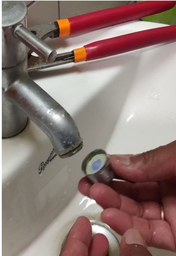
Water Aerator Installed in all
